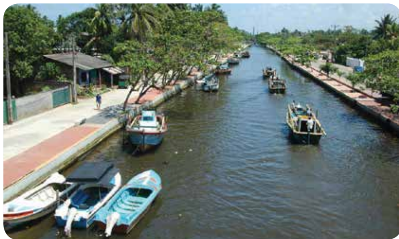
Rehabilitated Hamilton Canal
