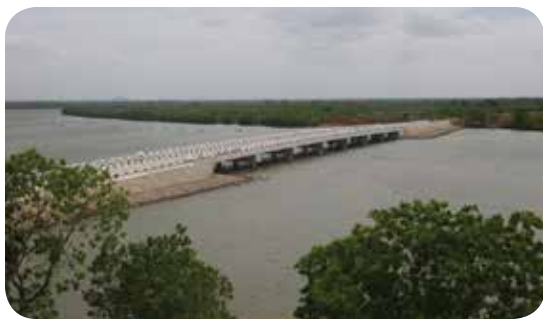
Panichankerni bridge and causeway
