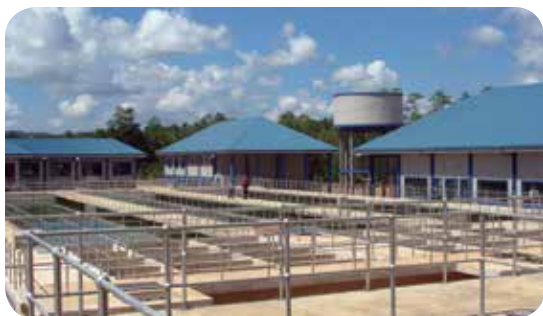
Water treatment facility at Moratuwa
