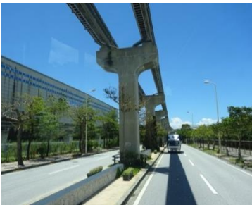
View of Simple Beam Structure
