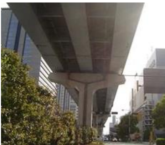
View of the Slab Structure
